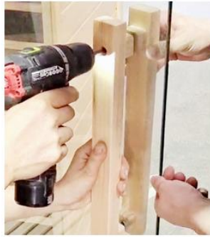
Door Handle Installation
